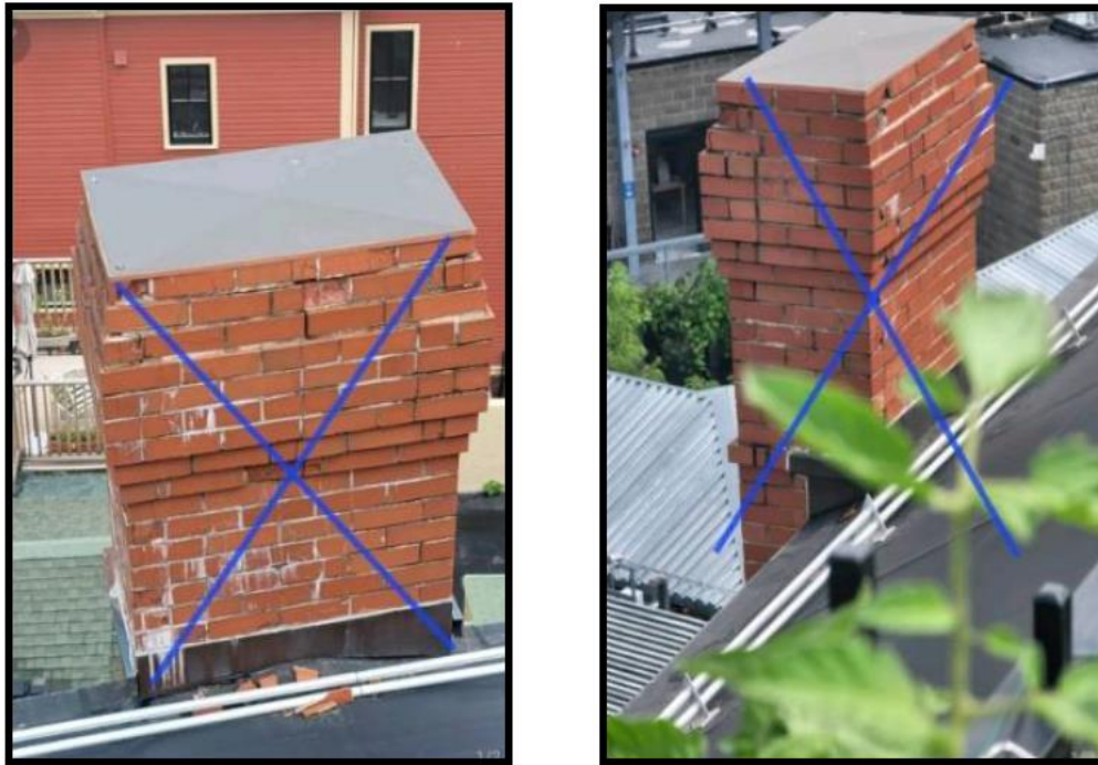
Above: Close-up images of the two chimneys on the left elevation proposed to be removed and reconstructed
