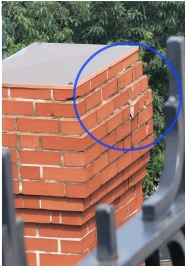
Stress cracking on chimney,
